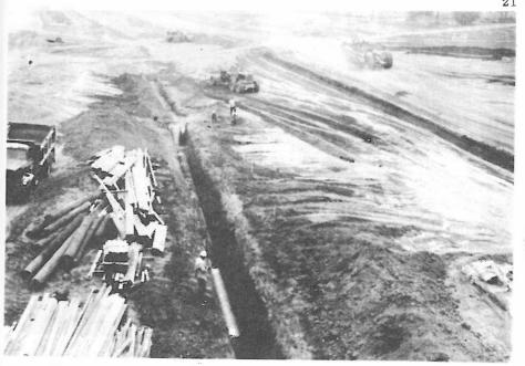
Daley workers are busy as beavers on eastbound lanes of I-8 at the Willows Interchange bridge. They are burying large culvert pipes, grading and banking, then the paving starts.
